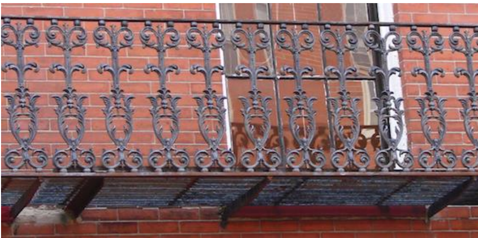
27 Monument Avenue balcony detail
