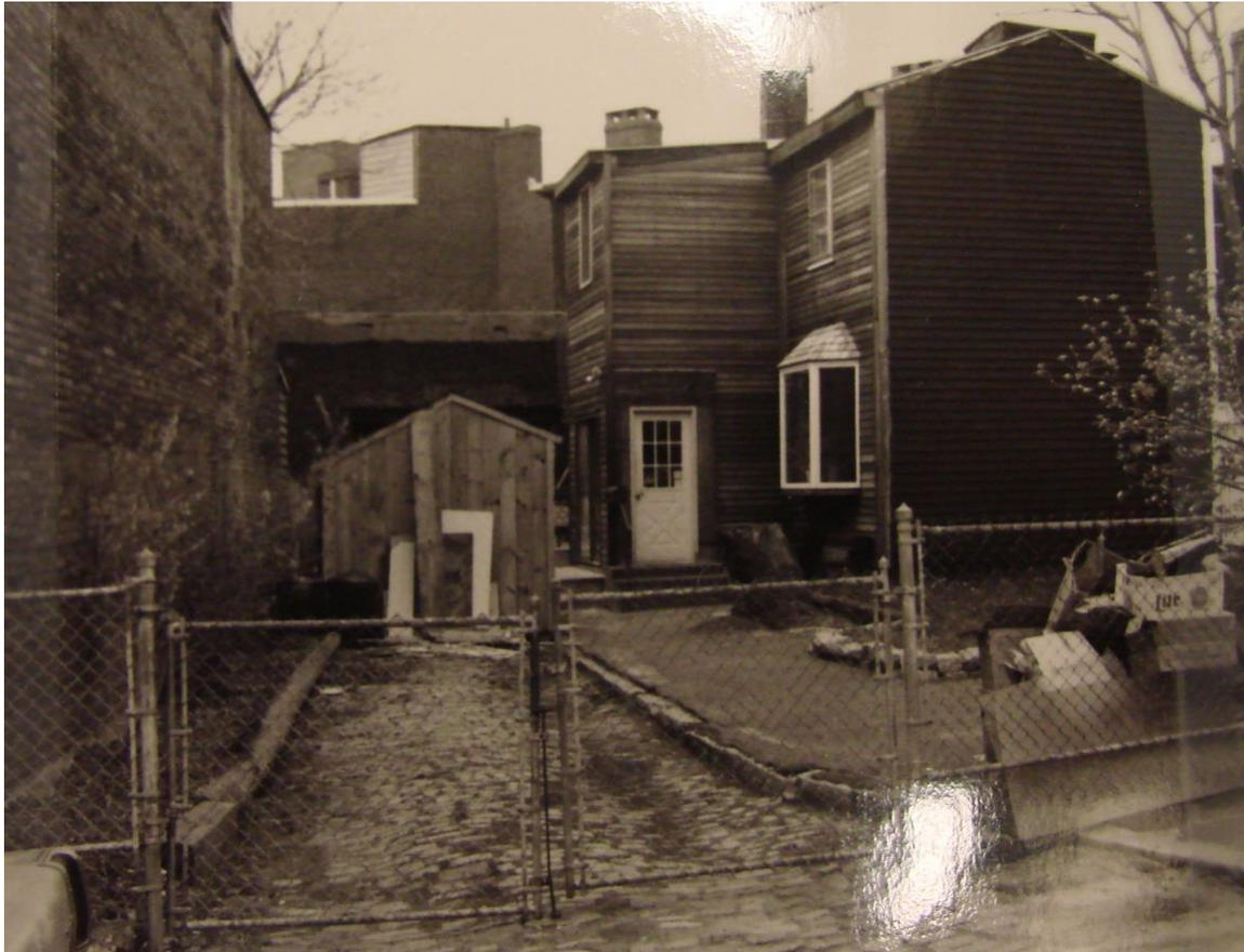
Number 10 Putnam Street is the rear ell of a two story, late 18th century house. It has been extensively reworked, and recently re-clad with clapboards, and a modern bay window addition. It has a low gable roof. Its edges are defined by narrow corner boards. The ell is missing its main block and the ell itself seems to have been rebuilt. It is set back from Putnam Street, facing a well-landscaped yard and borders on its southeast side a cobblestone a passageway of considerable age.
