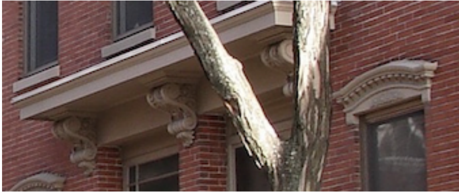
1, 3 Auburn Street entry, lintel detail 2015
