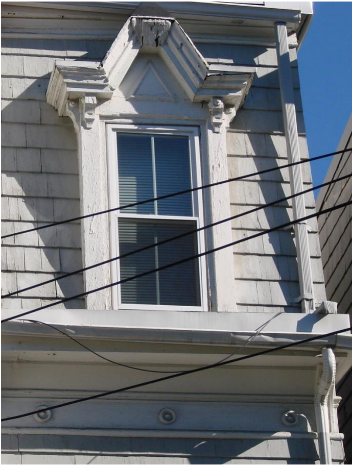
15 Lexington cornice and third floor window detail, 2015
