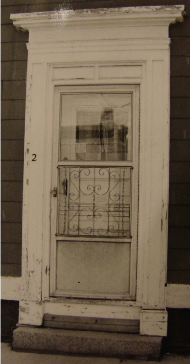
2 Salem Street Avenue entry detail
