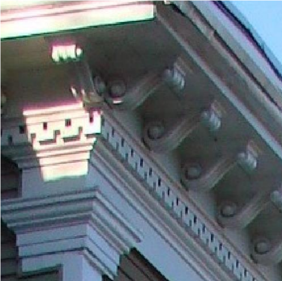
22 Trenton Street cornice detail
