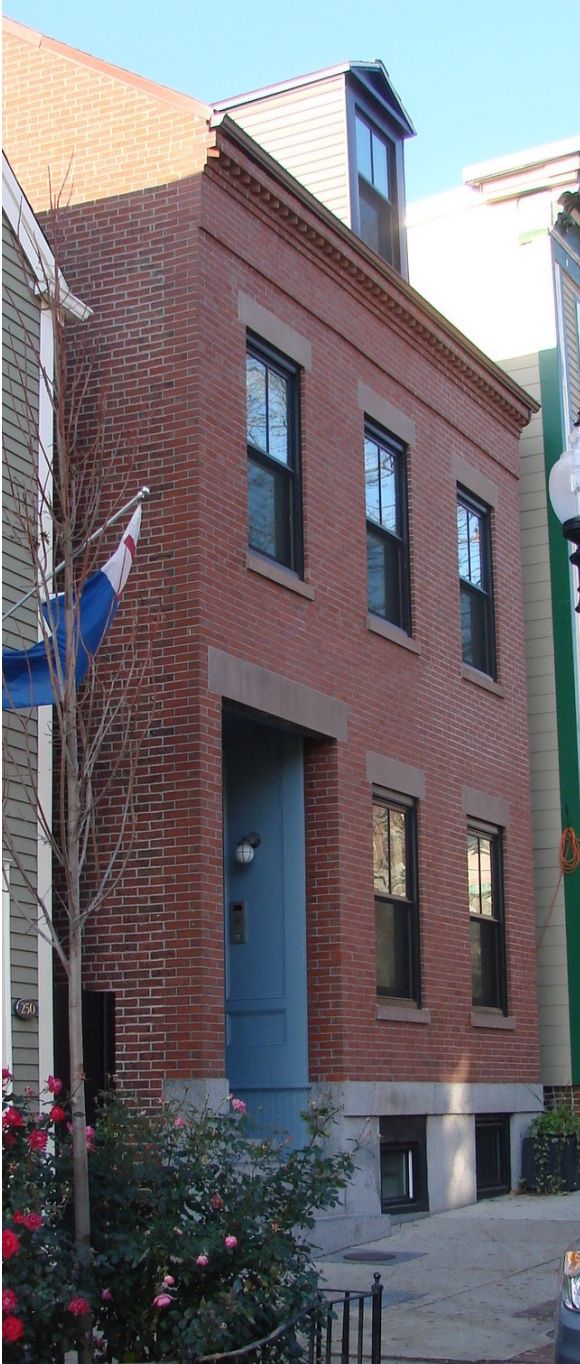
252 Bunker Hill Street
