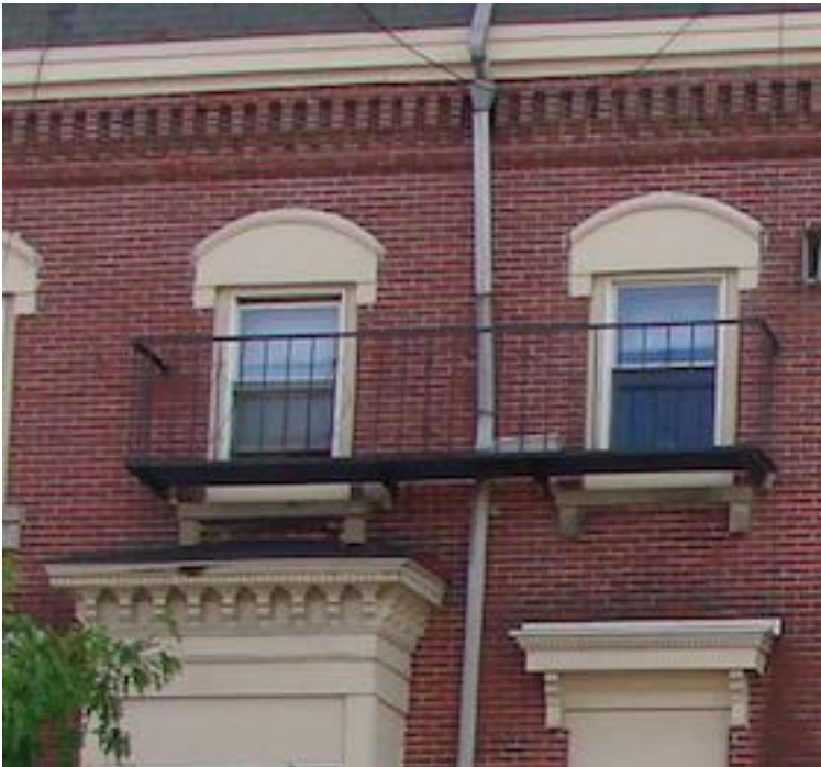
269 Main Street window, and cornice detail
