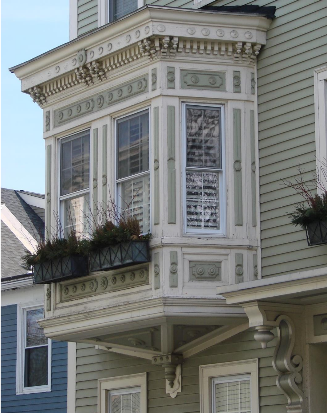
27 Trenton Street, oriel and scroll bracket detail
