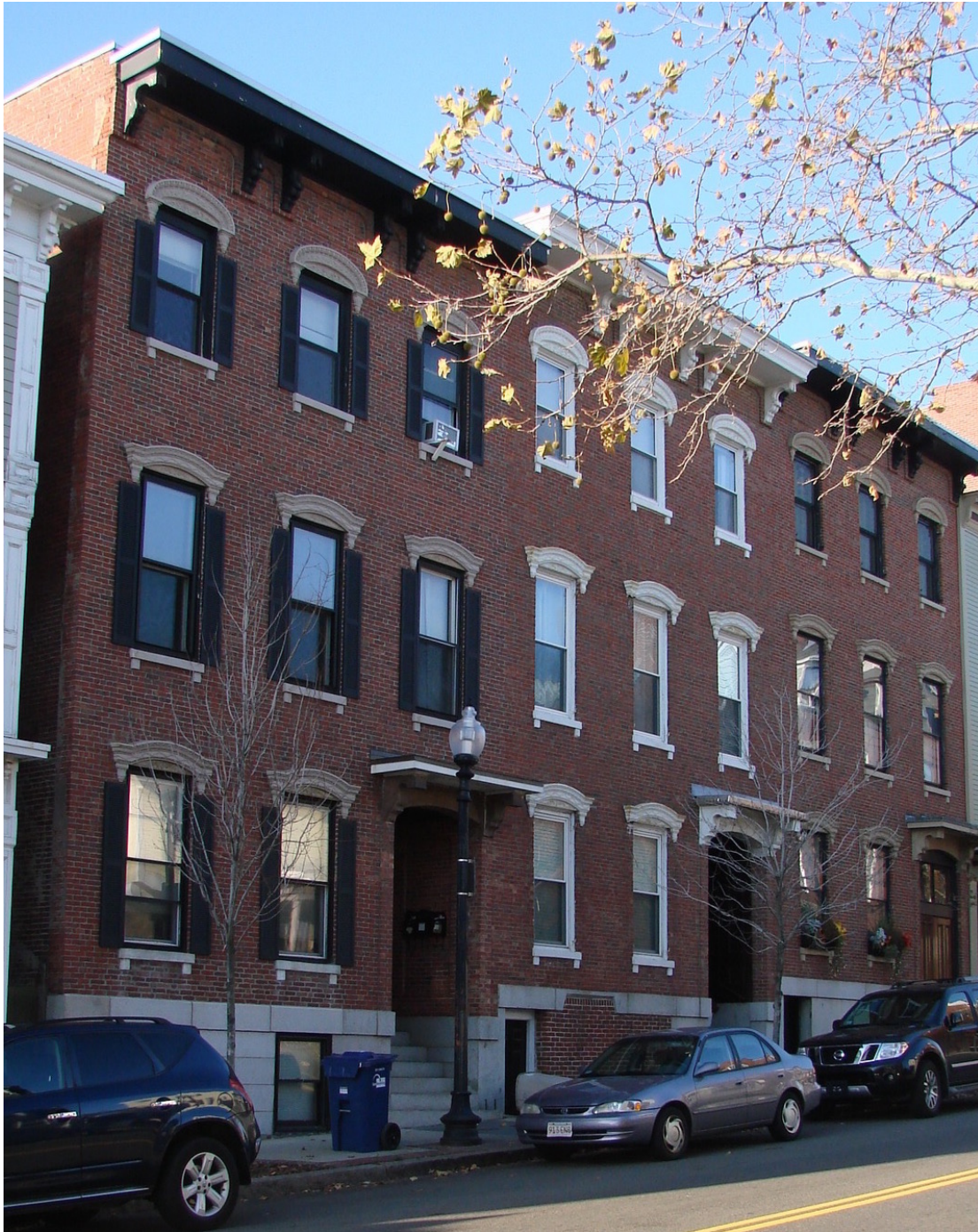
276-280 Bunker Hill Street
