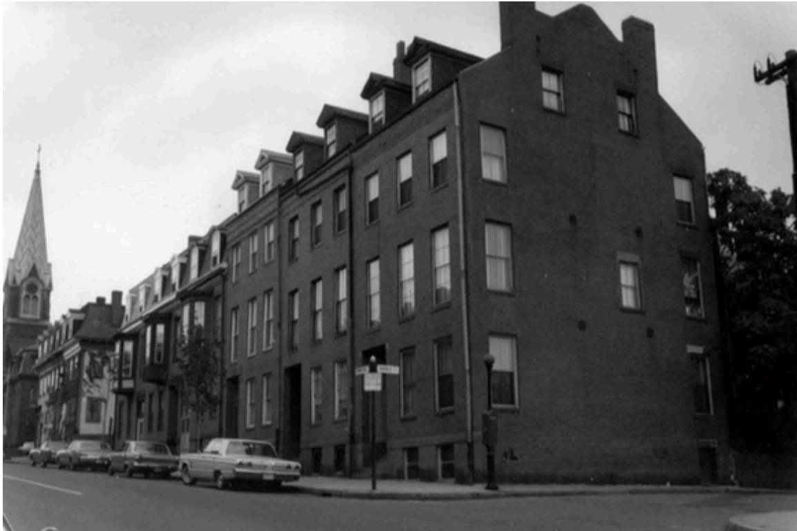
289-285 Bunker Hill Street
