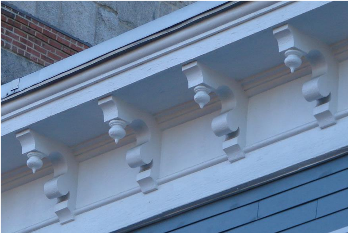
32 Winthrop Street cornice detail
