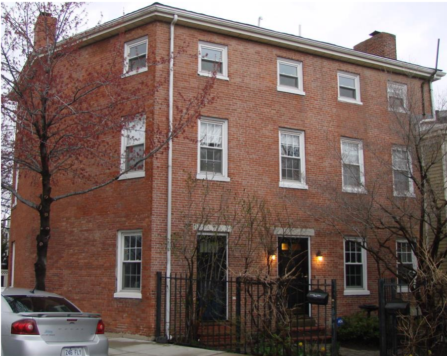
31 Union Street, southeast façade
