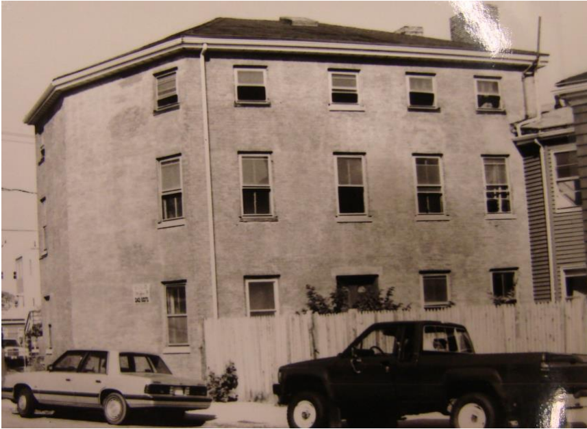
31 Union Street, southeast façade
