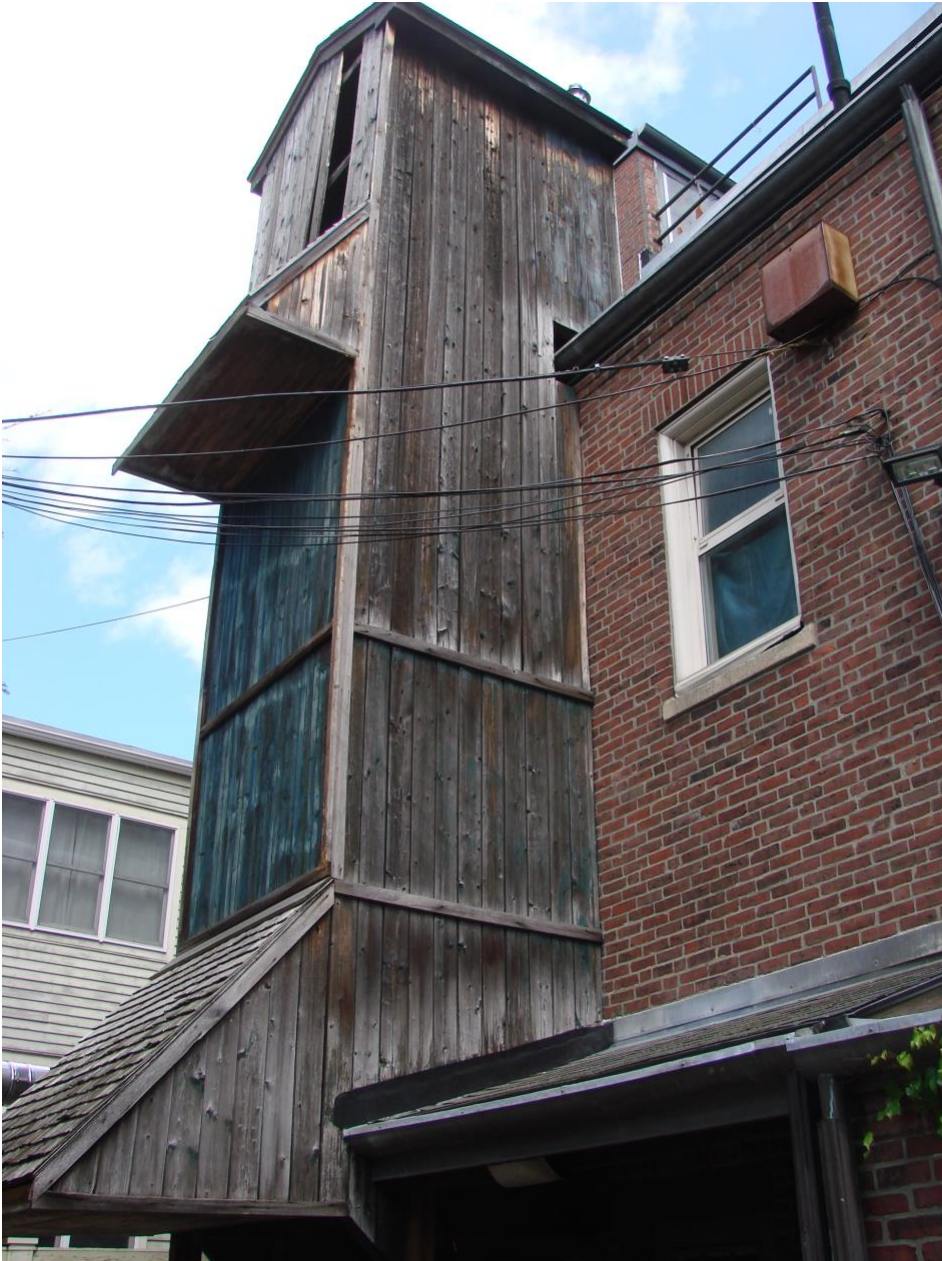
Rear wall hose drying rack, ? age, no longer in use
