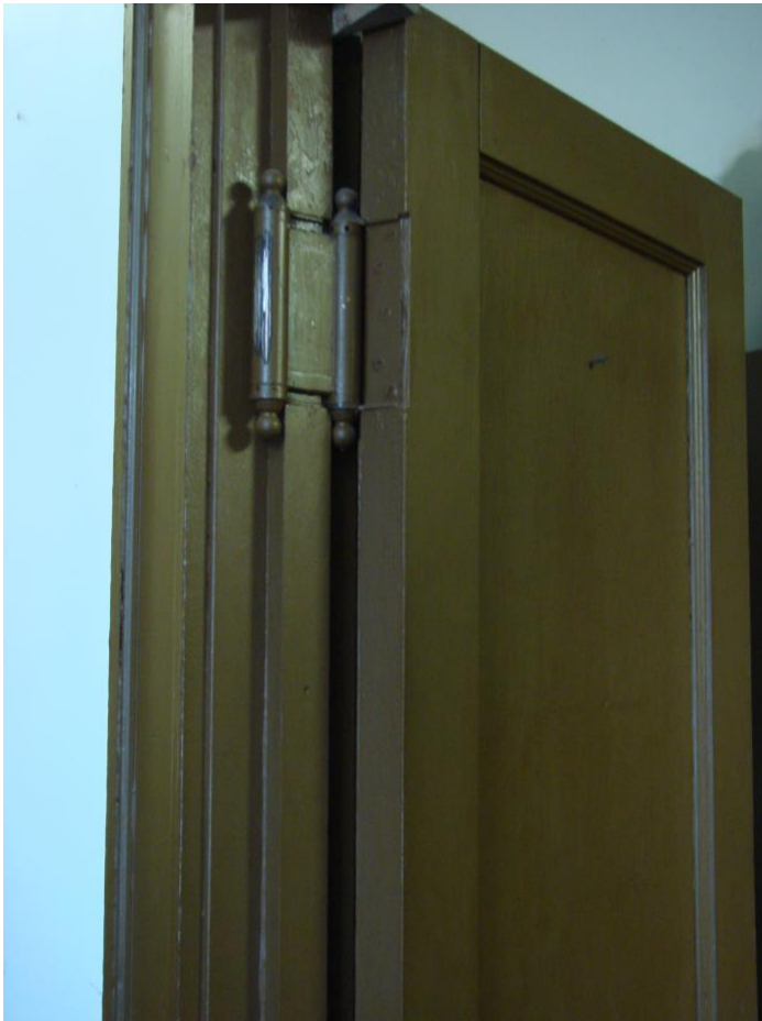
Second floor door, hinge, old section (1853)
