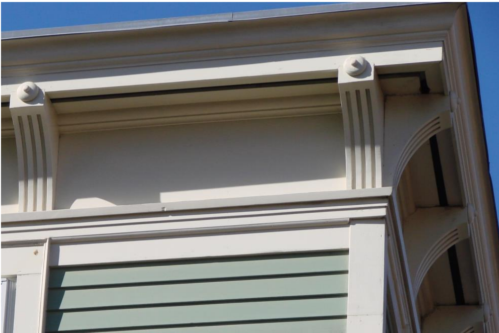
37 Winthrop cornice detail
