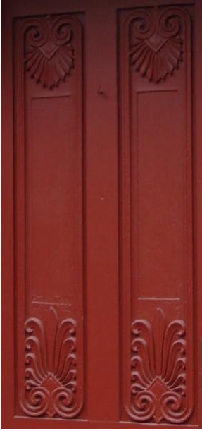
Stable door detail
