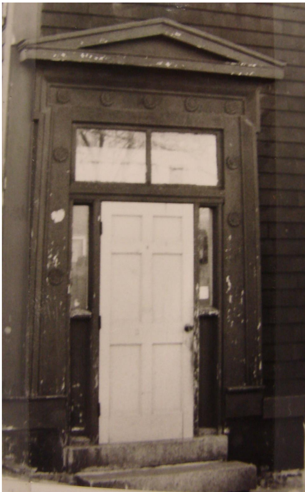
39 Mead Street entry
