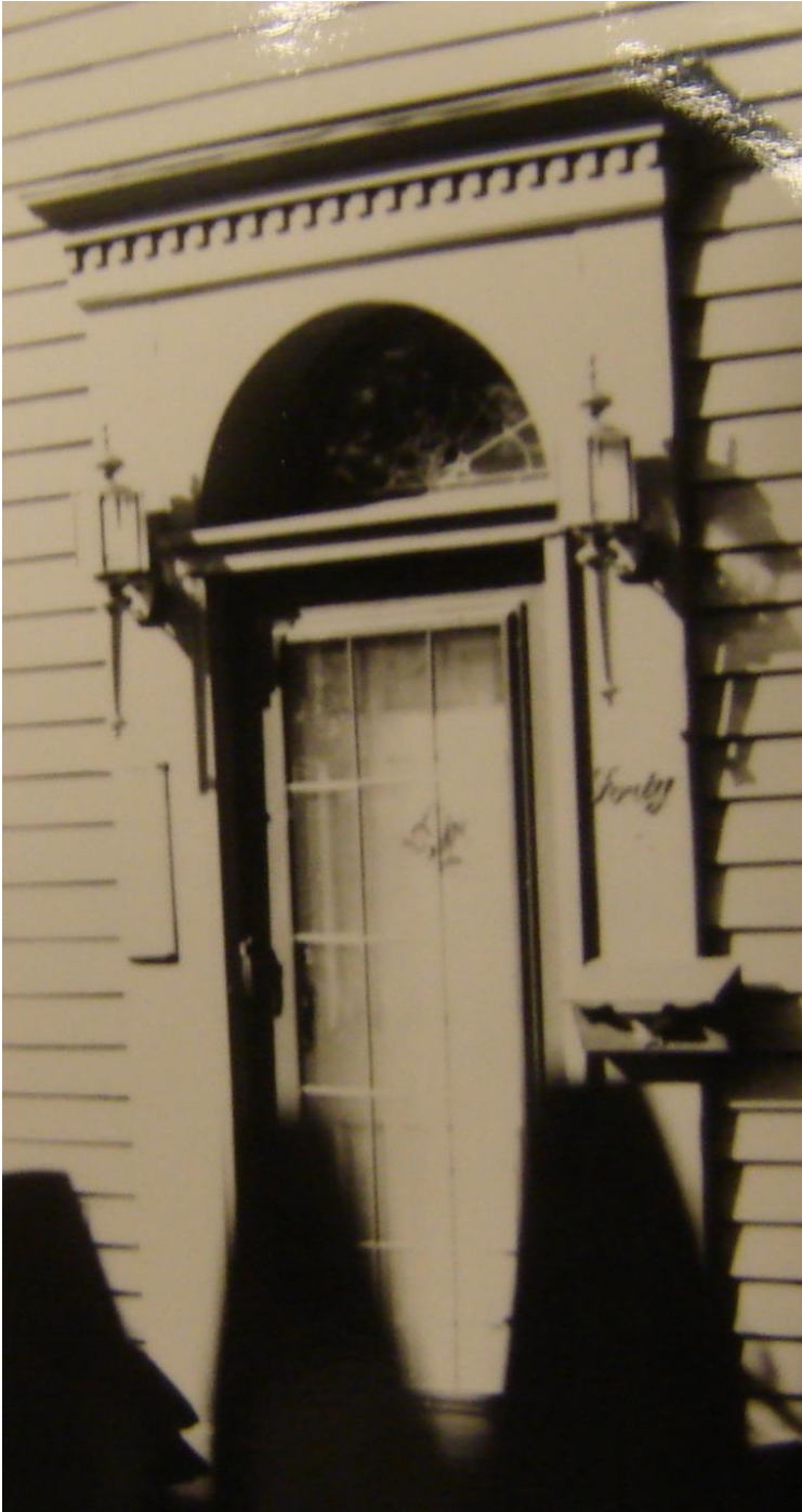
40 Washington Street, entry detail
