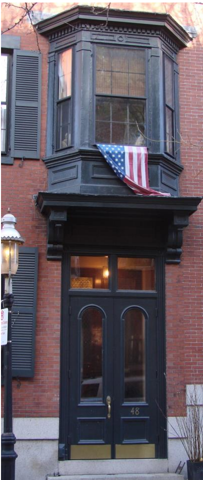
Entry, oriel, 48 Monument Avenue
