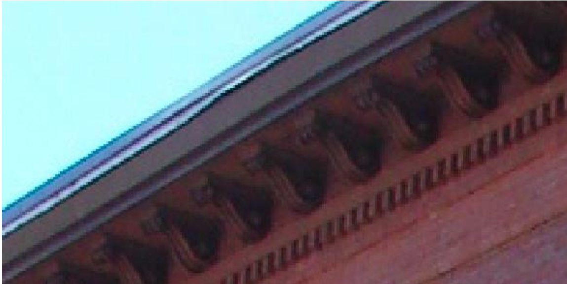
46 Mount Vernon Street cornice detail
