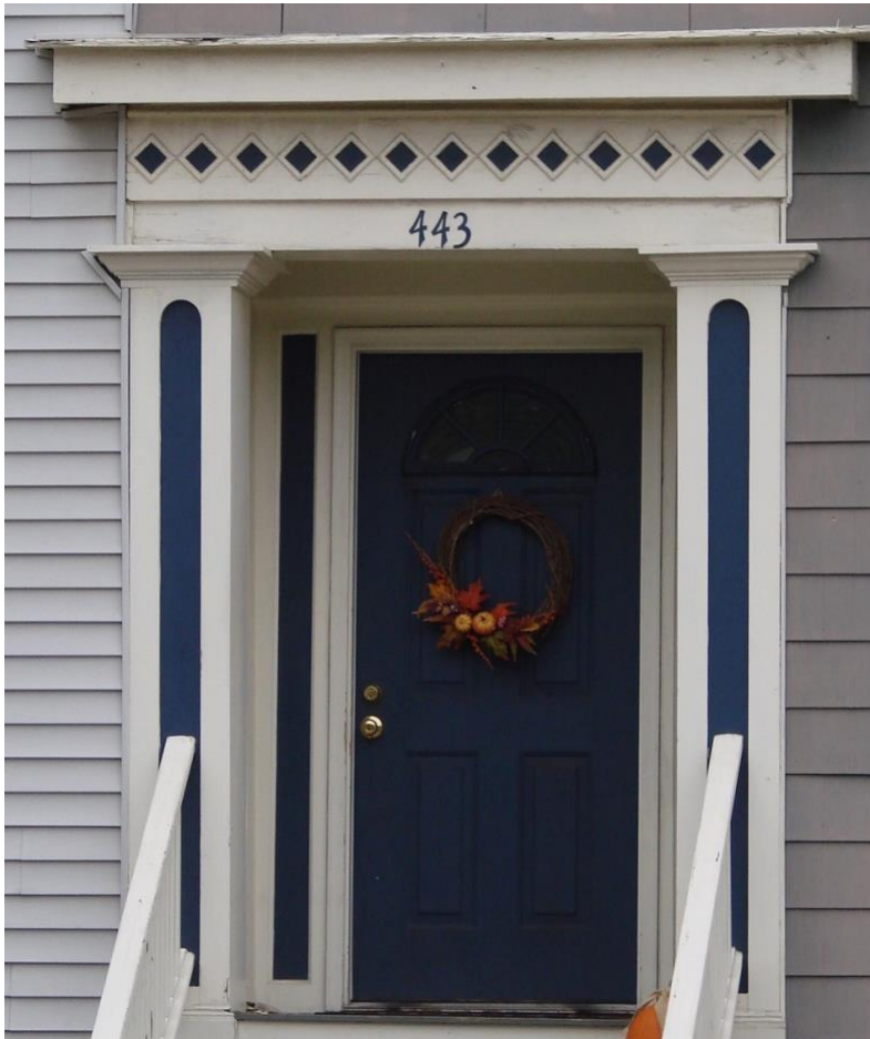
443 Main Street, entrance detail 2015
