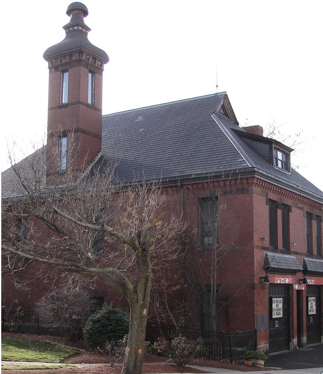
454 Bunker Hill Street
