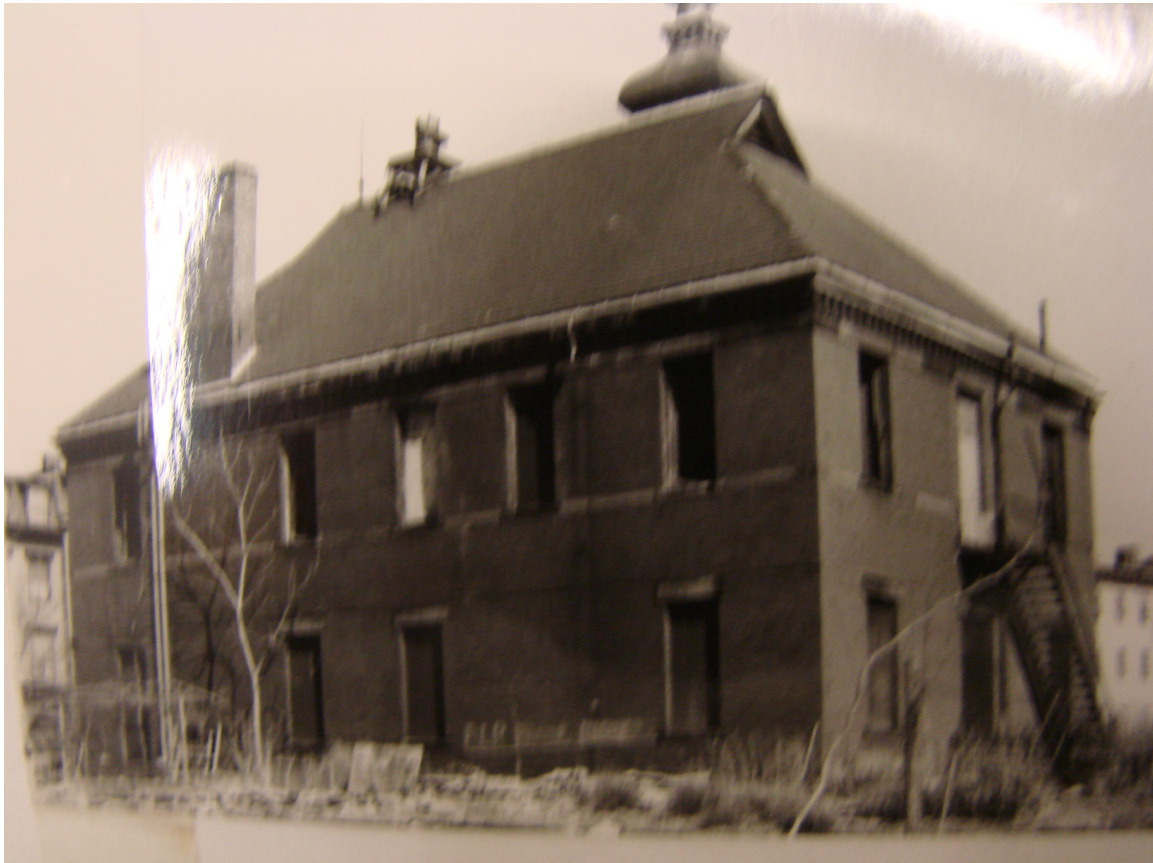
454 Bunker Hill Street
