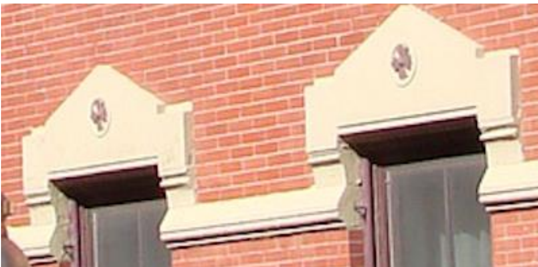
54 Monument Avenue first floor lintel detail 2015
