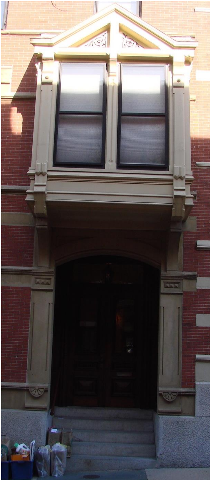
52 Monument Avenue, oriel, entry detail
