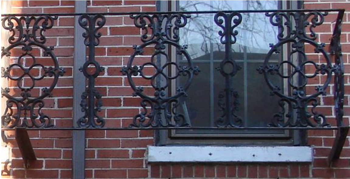
58 Elm Street balcony detail
