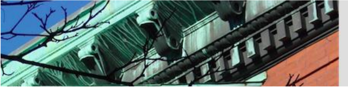
60 monument Avenue cornice detail
