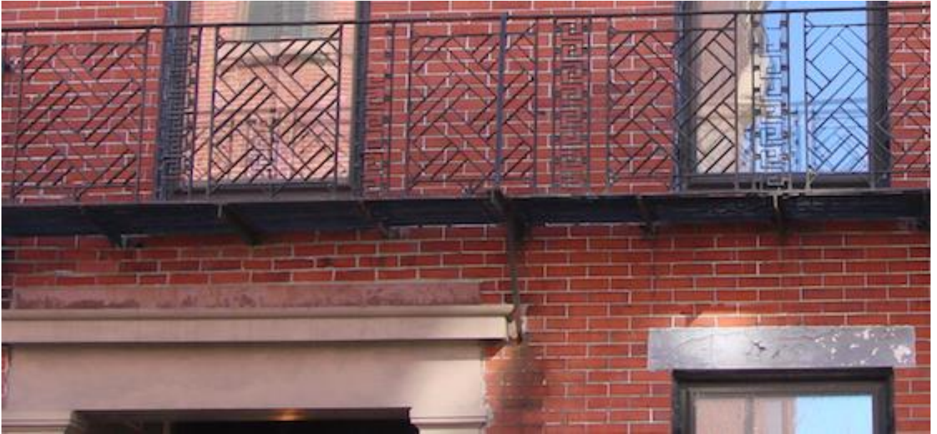
21 Harvard Street balcony detail
