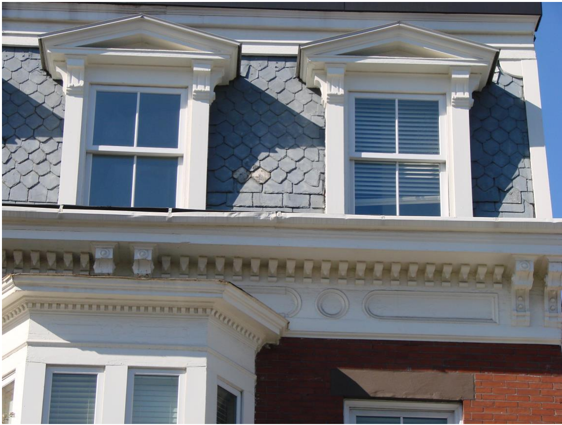
72 High Street Cornice, roof detail
