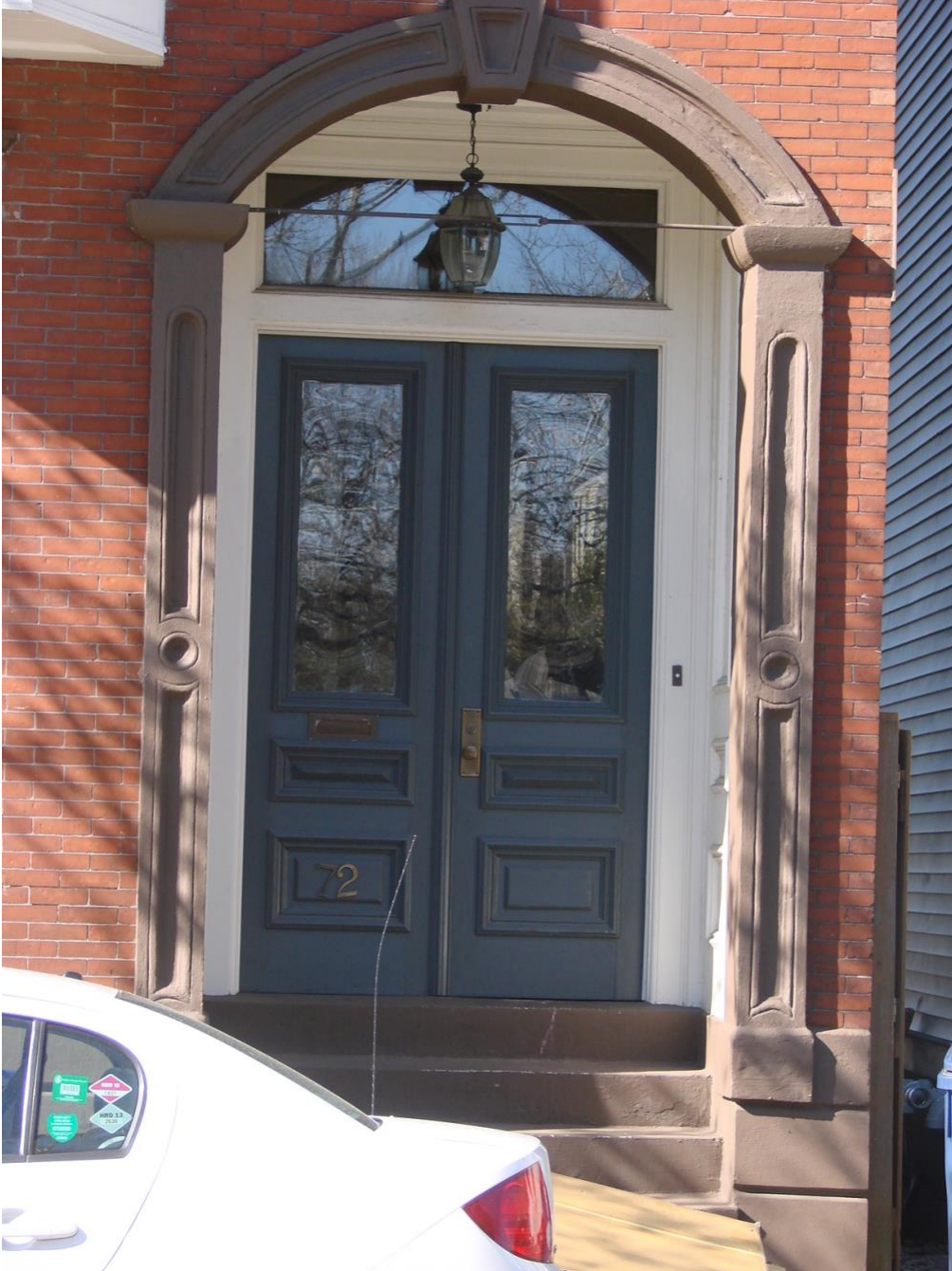
72 High Street entry detail
