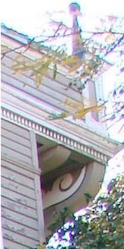
Parapet bracket, plinth, and finial detail
