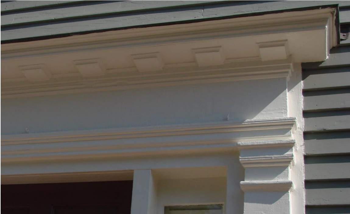
85 Warren Street entry detail
