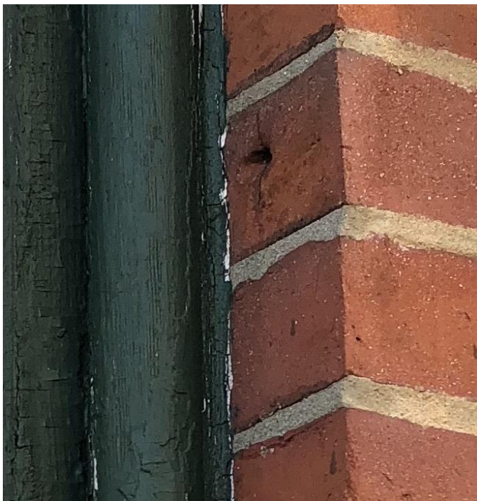
11 Union Street, window molding detail
