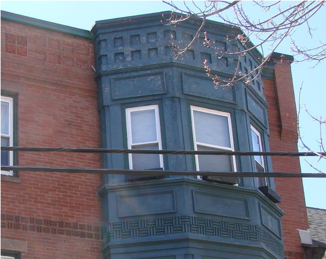
11 Union Street cornice and oriel detail 2015
